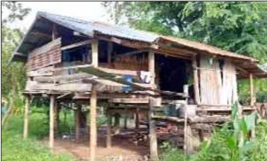
Figure 4: Typical of poorly constructed bamboo + corrugated zinc house.
