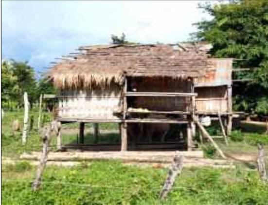
Figure 2: Typical of poorly constructed wooden + corrugated zinc house.
